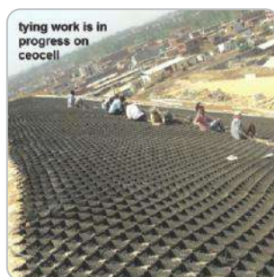
Tying Work of GeoCell
