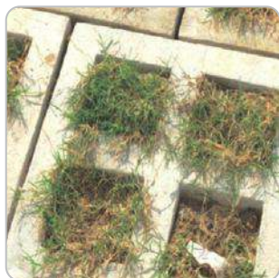
Grass Paver Block installed
