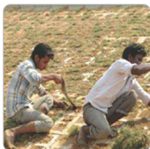
Installation of Grass Paver Block
