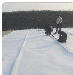
Installation of Geo-textile
