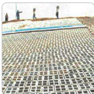
Laying of Grass Paver Blocks
