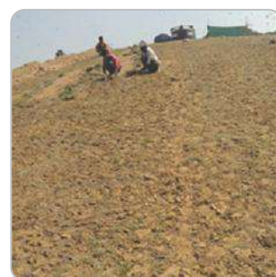
Laying of Top Soil (Vegetation Layer)
