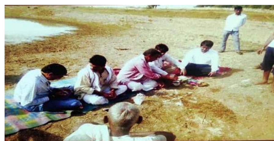
Gram Panchayat Bhatri site before digging work started
