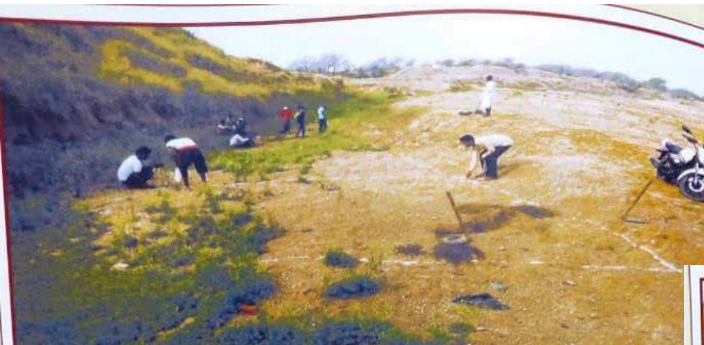
Gram Panchayat Sardhua site before dredging work started
