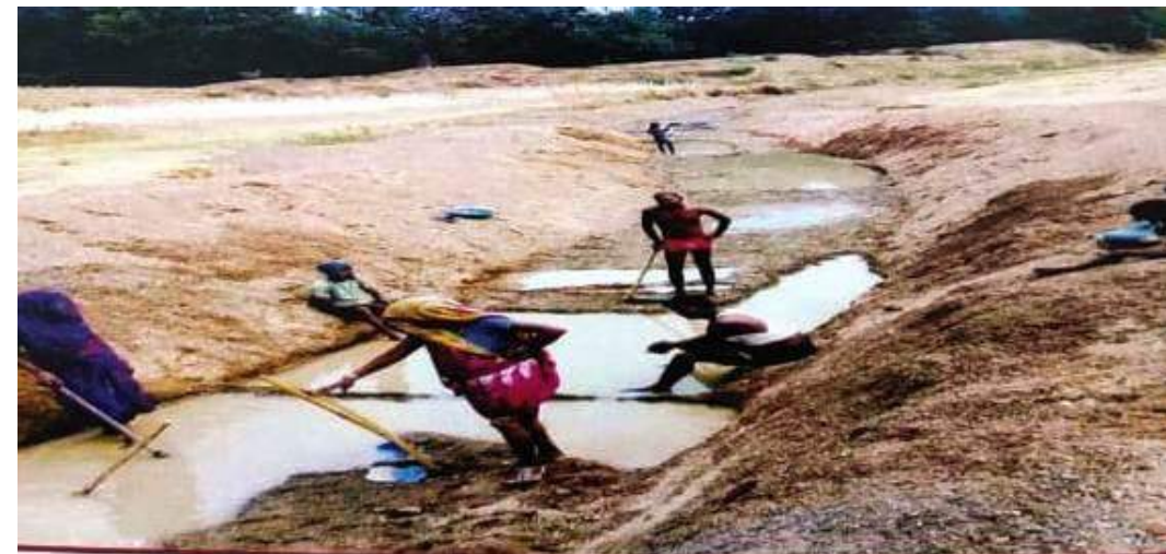
Start of water flow in river after dredging
