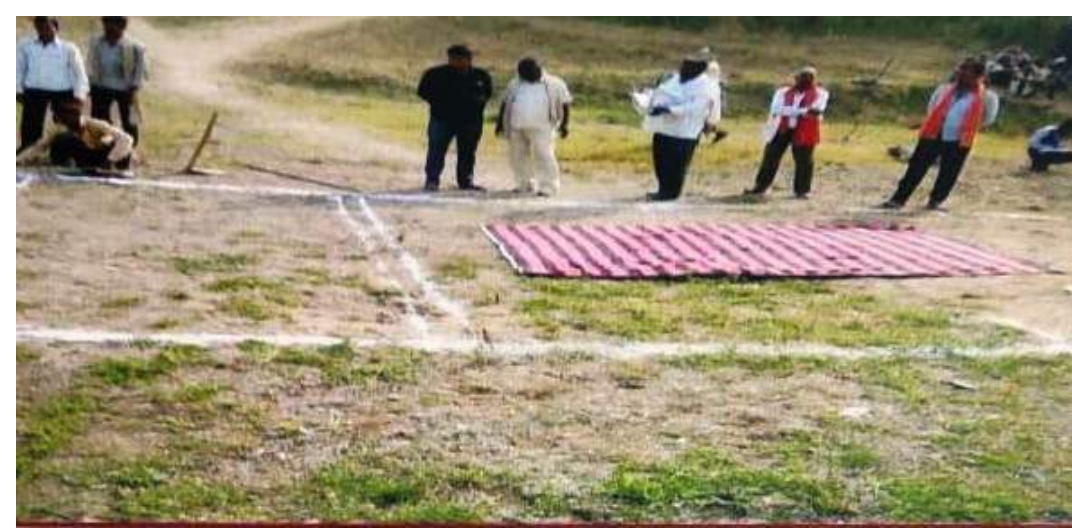
Gram Panchayat Arki site before dredging work started
