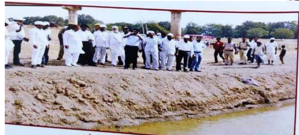
Start of Water flow after completion of work
