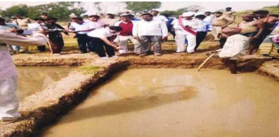
Inspection by District Magistrate after completion of work
