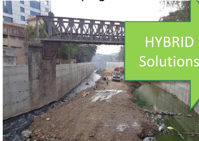
Routine desilting of rivers & nallahs
